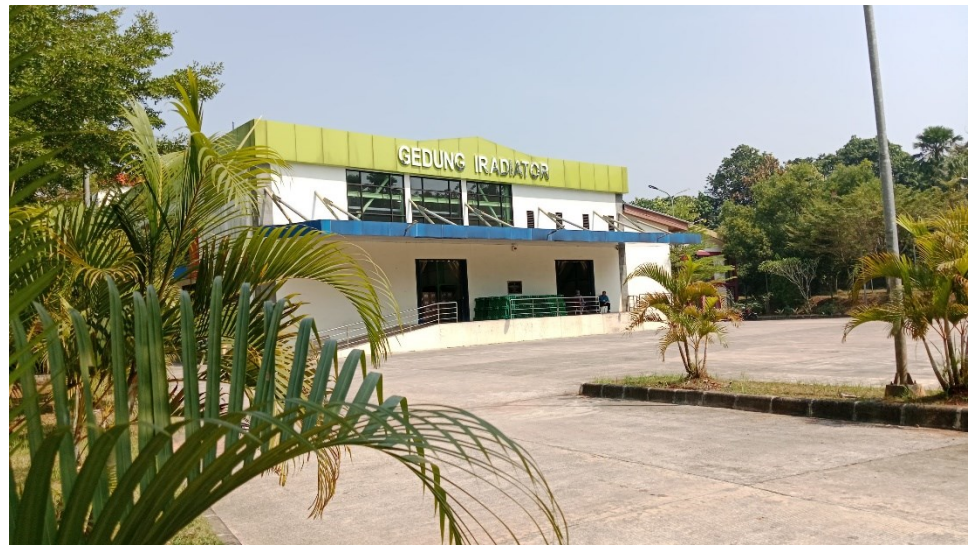
Figure 1. Exterior view of the gamma irradiator pilot project facility.
