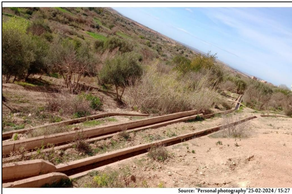
Image 1. Cement water channels for water transport in aghbal community.
